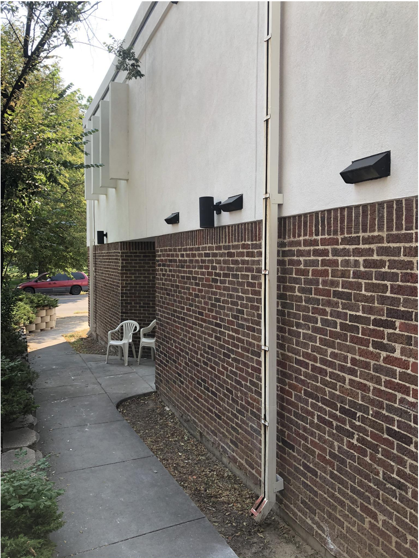
5. NORTH FACADE (1 OF 2)
