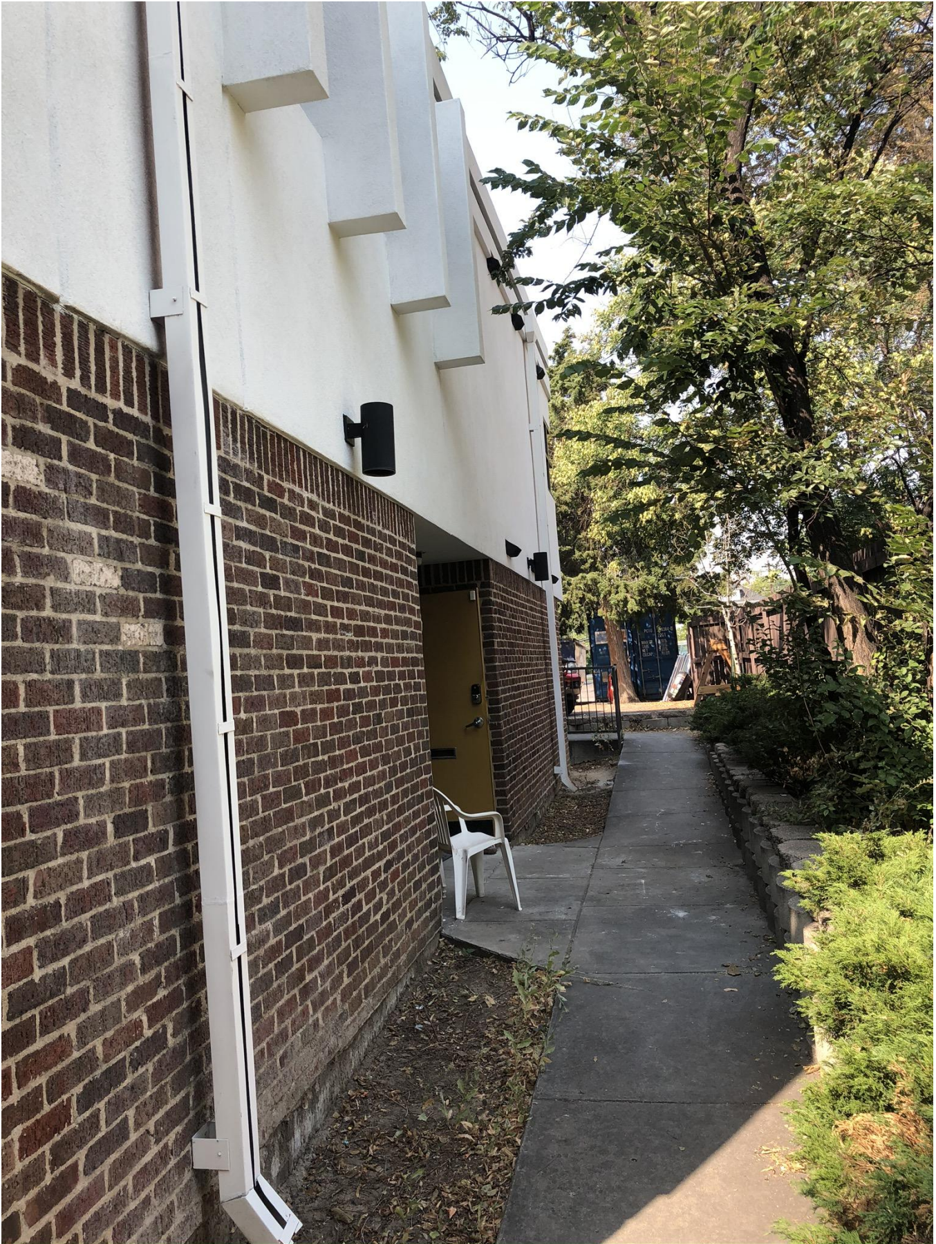
6. NORTH FACADE (2 OF 2)
